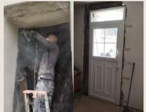
Chantier PO COB (29)
